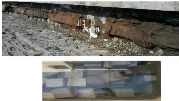
Fig.6 Curing of concrete blocks & beams
