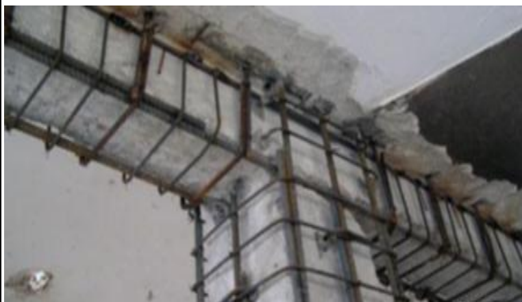
Photo. Strengthening of beam
