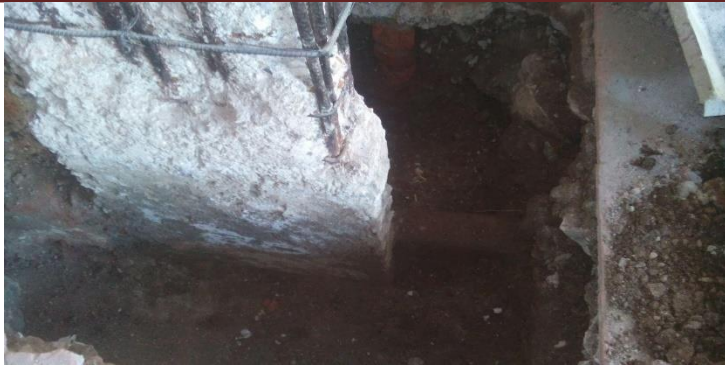
Photo. Excavation around the footing
