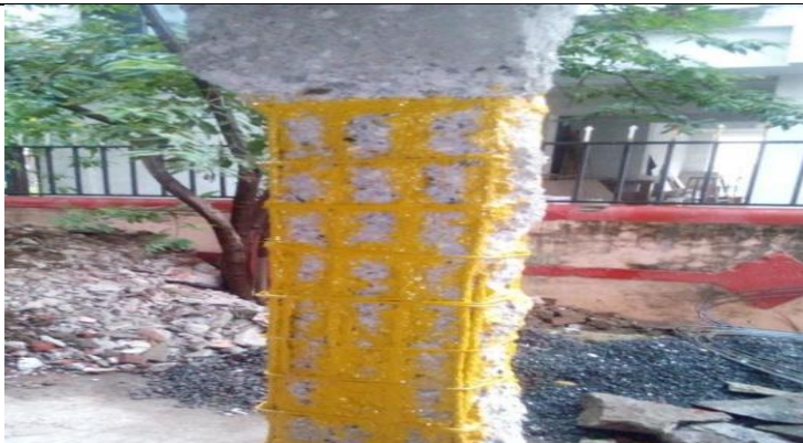
Photo. Column bars paint epoxy material (b)
