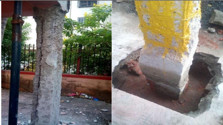
Photo. Column support by Jack
