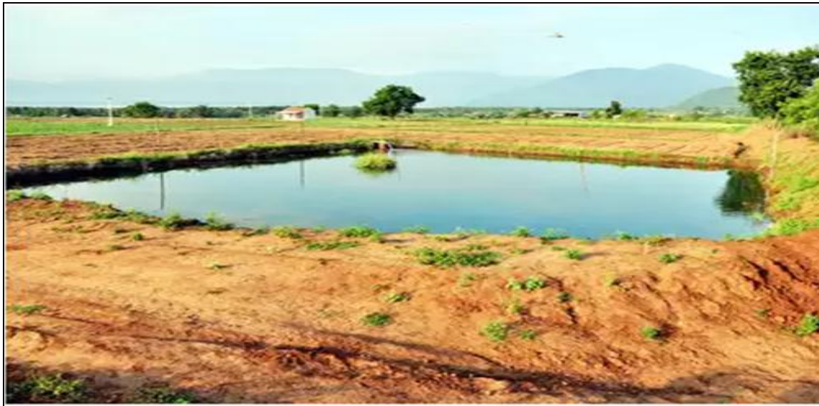
Figure no. 5.4 percolation tank
