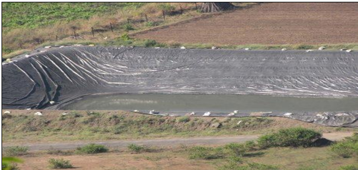
Figure no. 5.3 farm pond water harvesting
