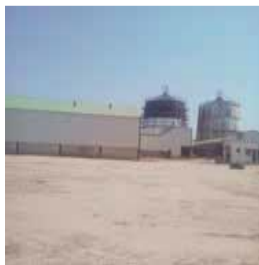
Picture 6: Overview of Biogas Plant
