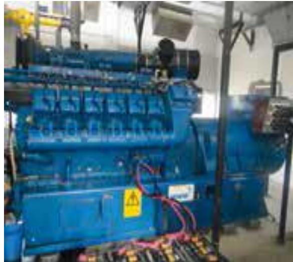
Picture 7: Electricity Generation Unit Along with Hydrogen Sulphide Scrubber
