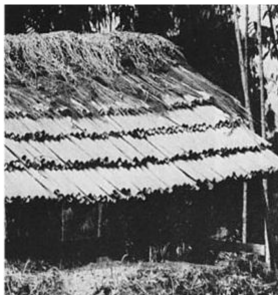
Fig 5(a) Double layers of bamboo shingles
