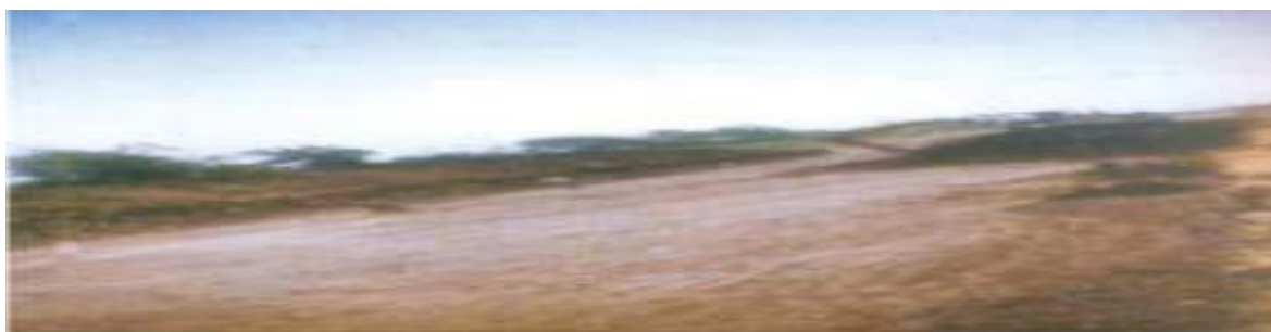
Figure 3: Construction of Road Embankment with Cohesive Non Swelling Soil (Moorum)
