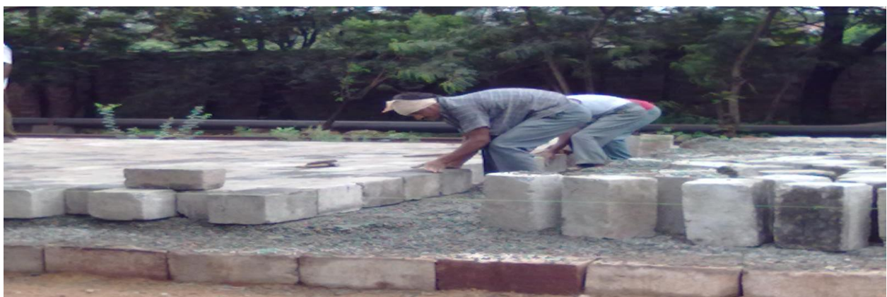
Fig. 23 Paving of C.C. Blocks
