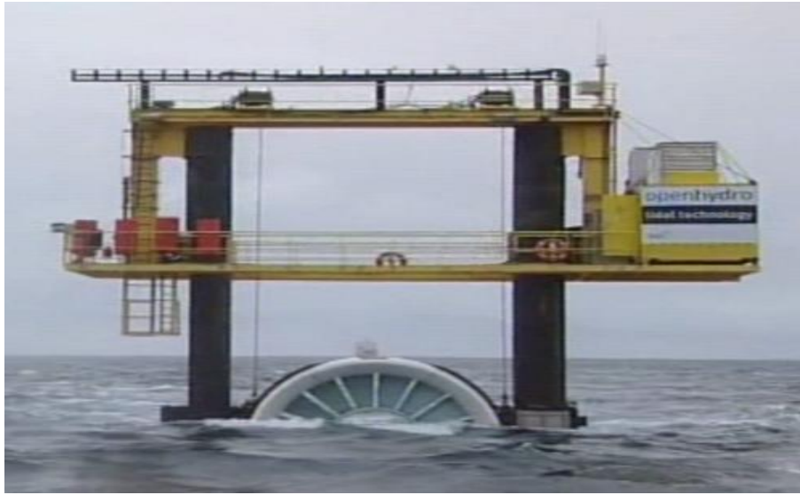
Underwater windmill under maintenance process.
